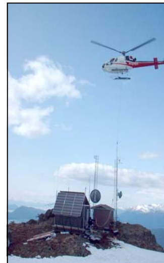
A helo drops ALMR Batteries on Saddle Mountain near Juneau
